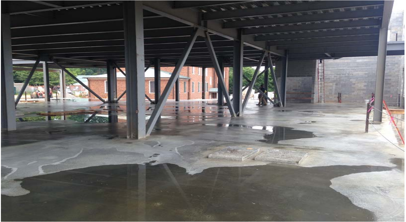
July 5, 2017 Ground Floor Slab
