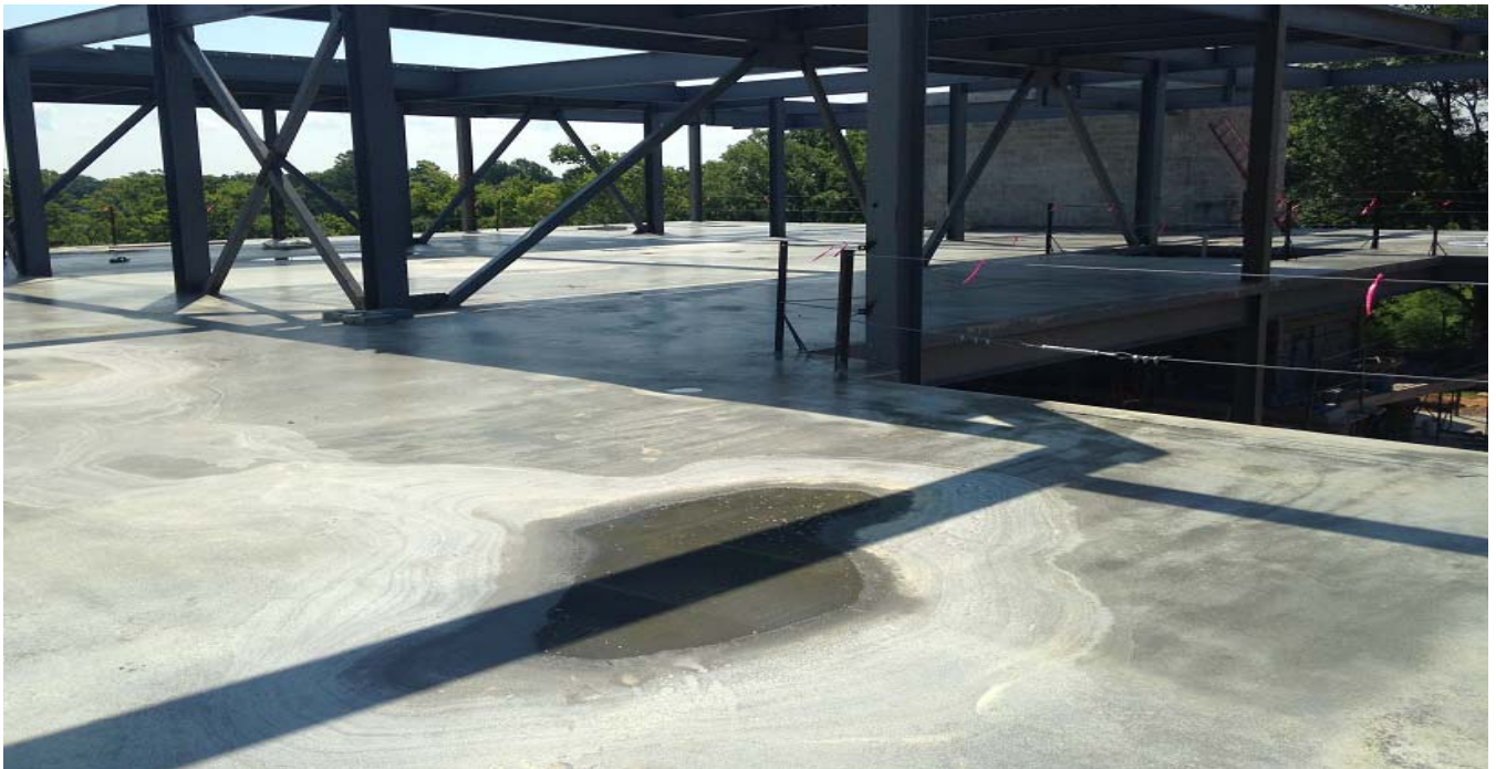
July 10, 2017 Upper Level Slab
