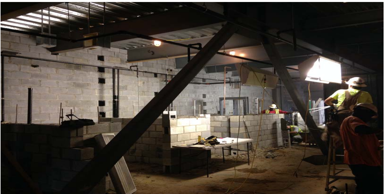
August 31, 2017 Lower Level Holding Cells
