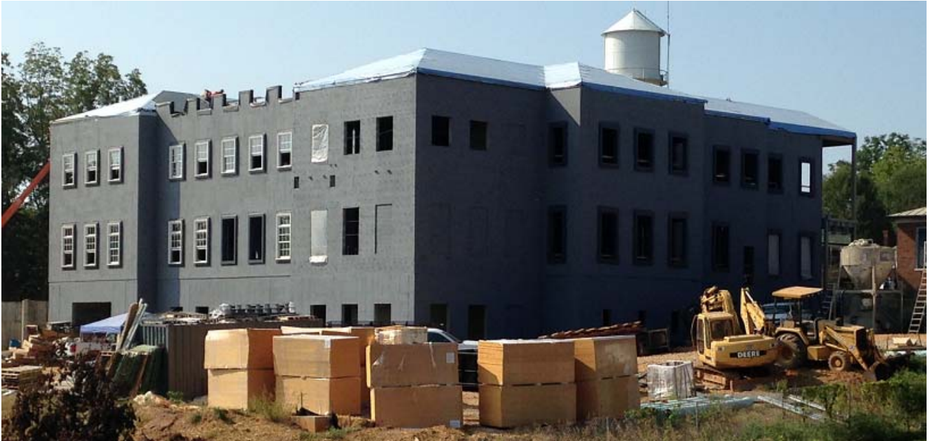
September 28, 2017 Northeast Corner Elevation
