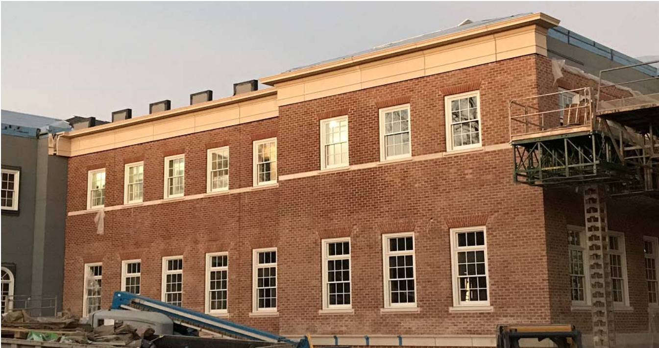
November 27, 2017 Southwest Corner Elevation
