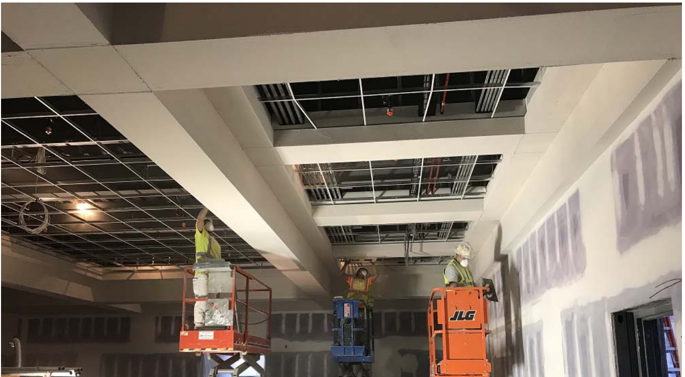
November 22, 2017 Ground Level Courtroom Plaster
