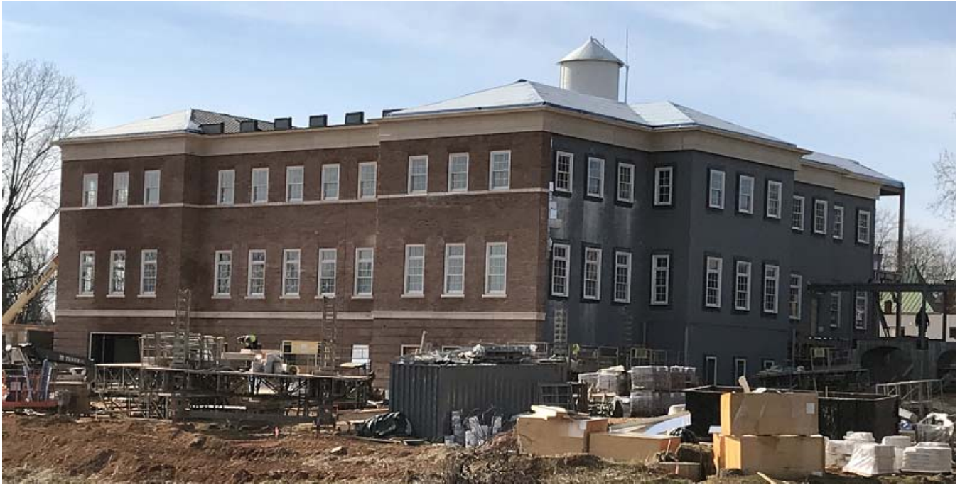
December 22, 2017 Northeast Corner Elevation
