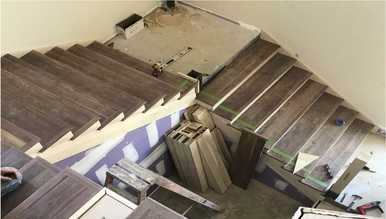
January 31, 2018 Public Stair
