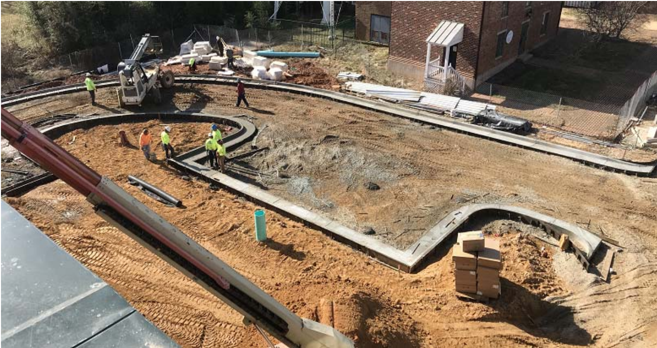
January 26, 2018 West Curb and Gutter
