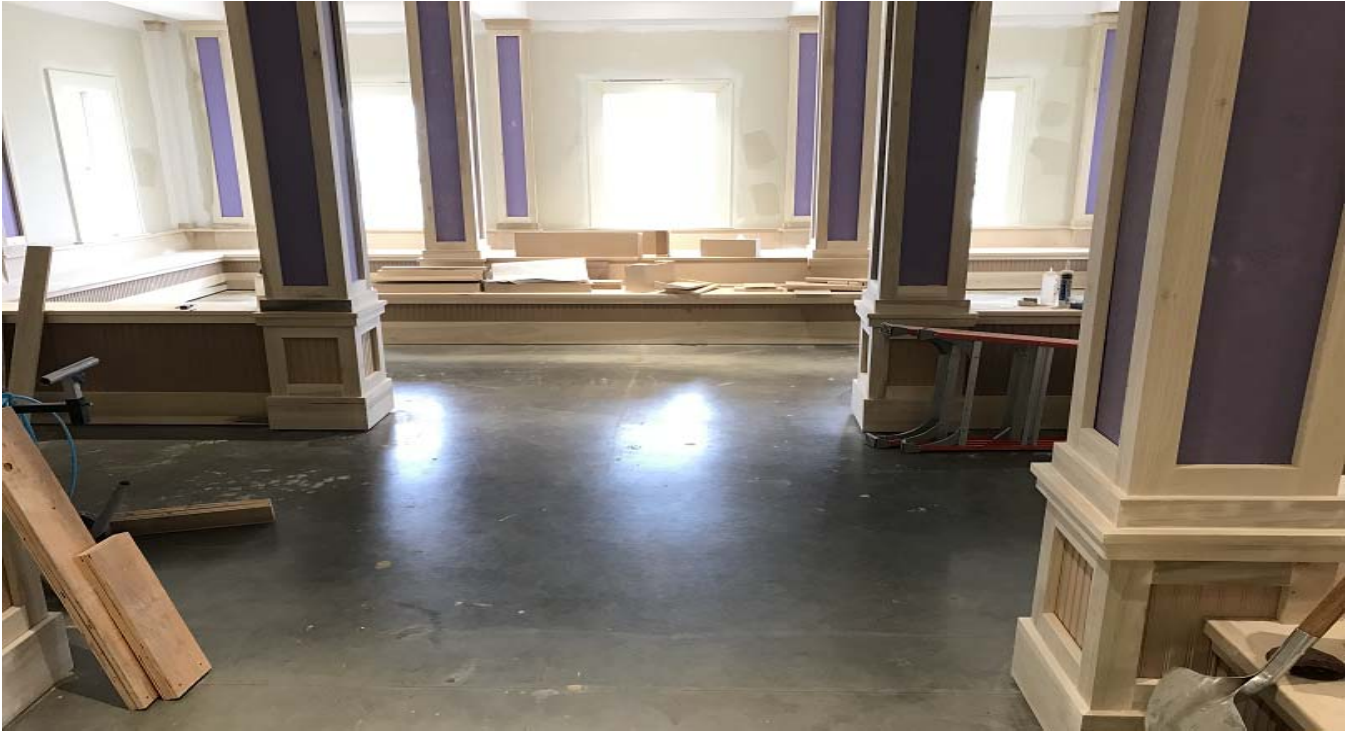
February 23, 2018 J&D Waiting Area Looking From Courtroom
