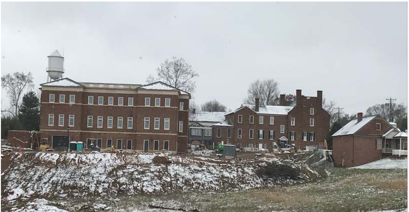
March 21, 2018 South Elevation from Route 40
