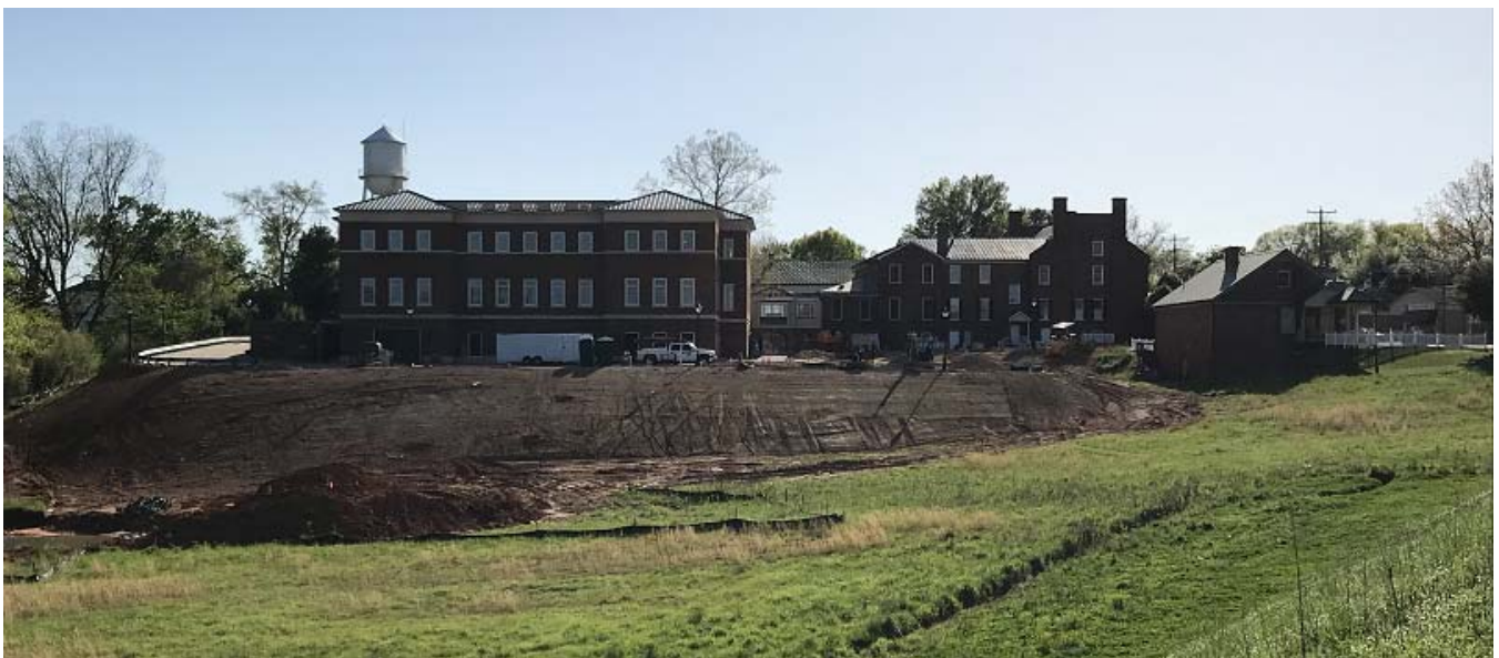
April 30, 2018 Looking from Route 40
