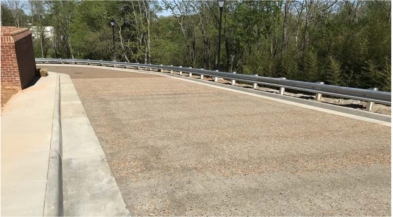
April 30, 2018 South Side Drive Exposed Aggregate Concrete
