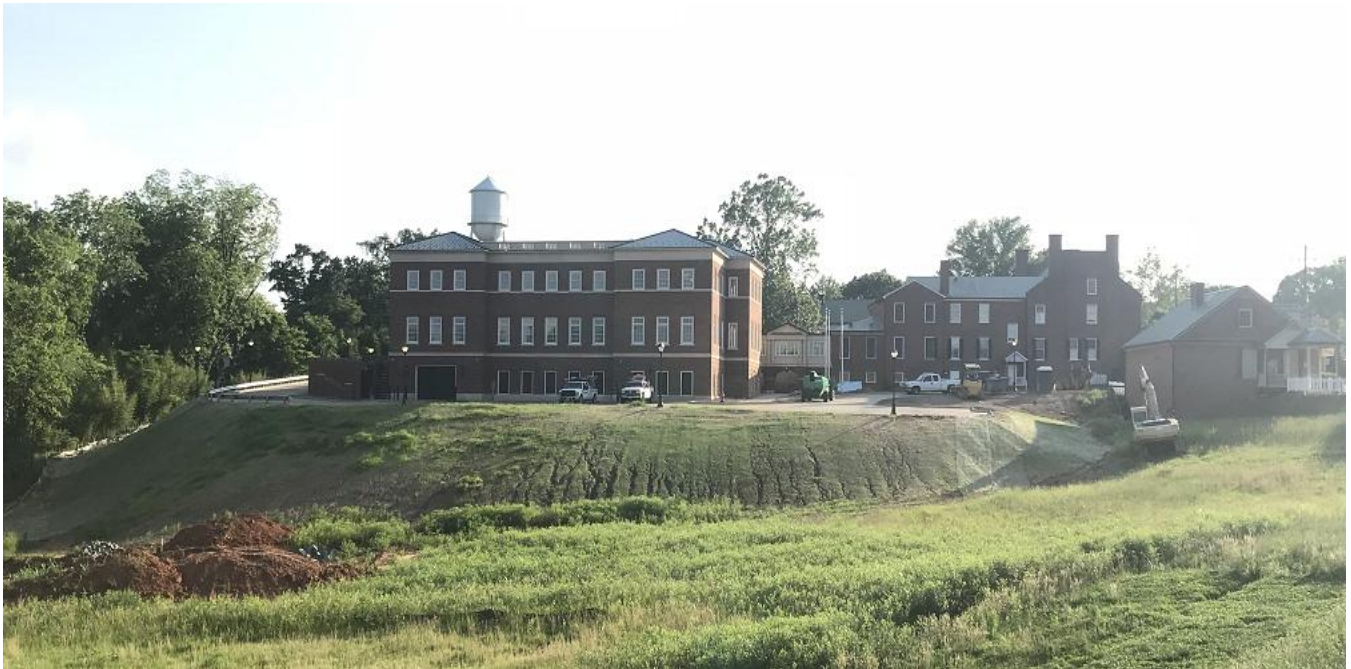
View of Rear of Building from Route 40 May 31, 2018
