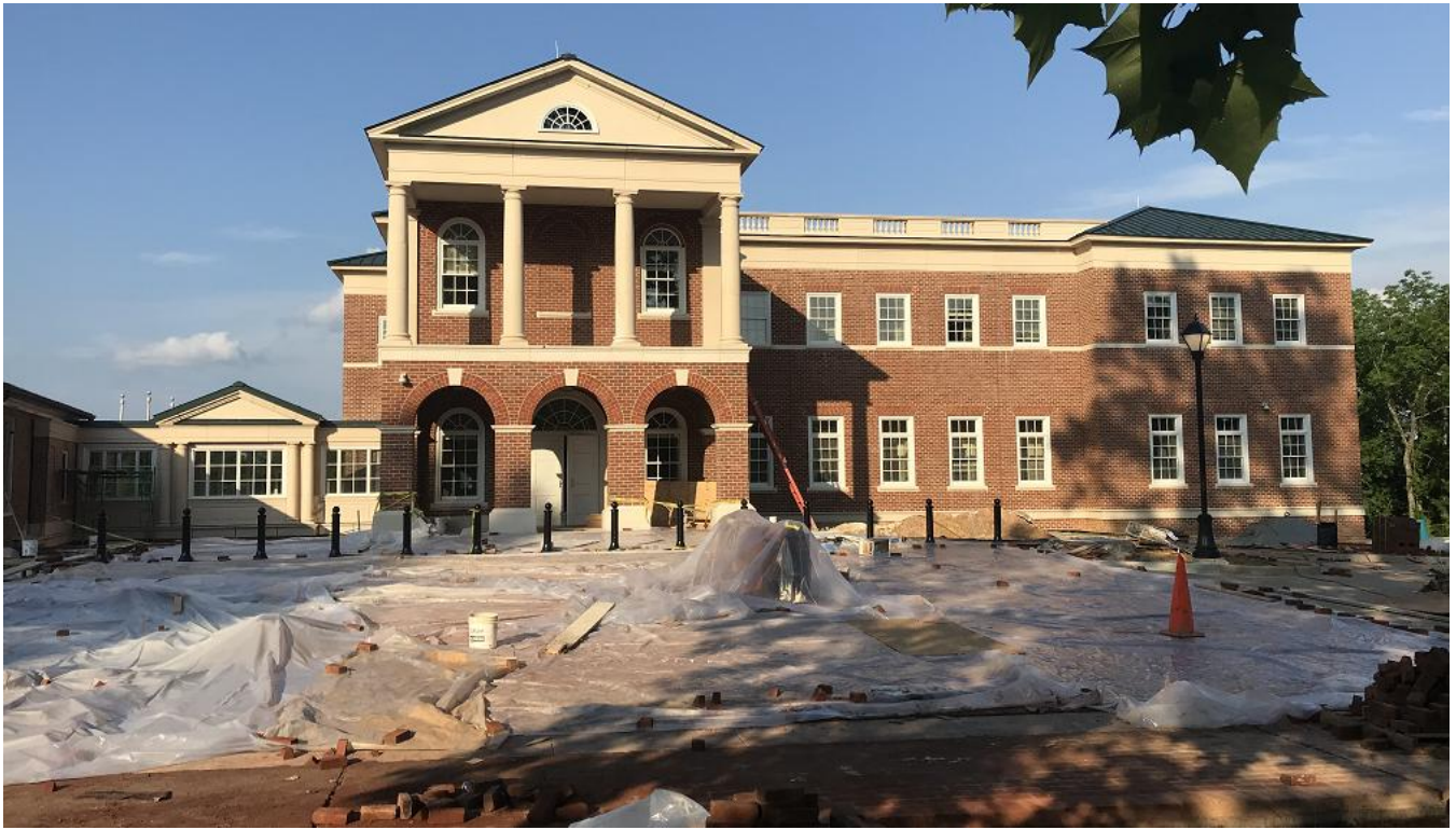
Front Entrance May 31, 2018
