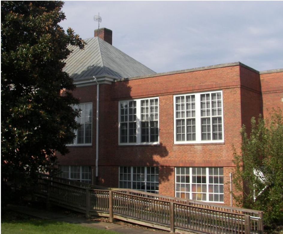
Sideview - STEPS Headstart Facility
