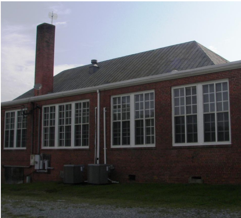
Rear & Opposite Sideview - STEPS Headstart Facility
